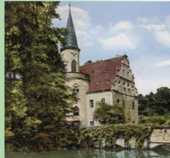
View of the south side of the castle with the filled moat and the mounted tower – this is how the castle could look in the future
